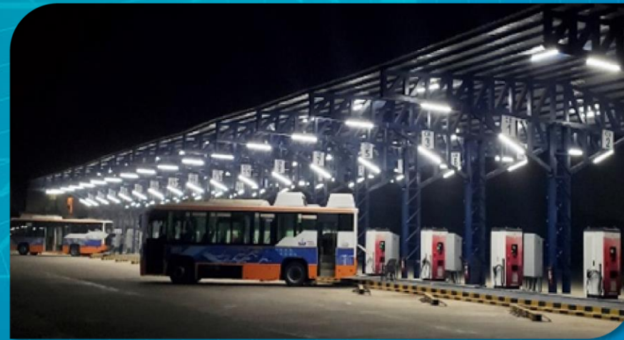
Fast charging depot
